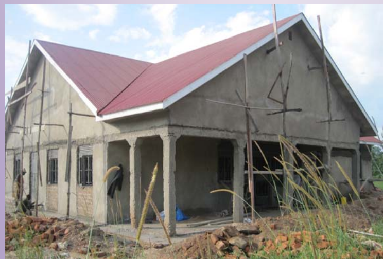
Above: Romogi Health Care Centre (PHCC) under construction
