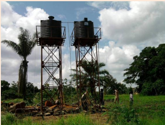
Two water tanks of 5000 litres each installed
