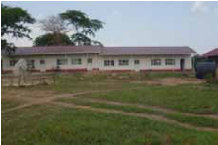
Classroom Block 2 - to be opened.
