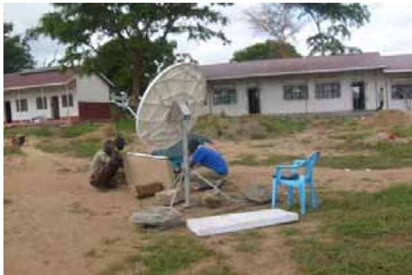
Installation of the Vsat. internet
